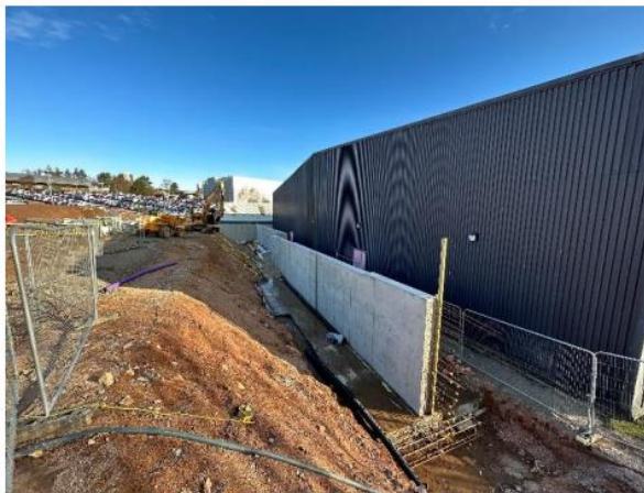
Grid Line BB East Side
