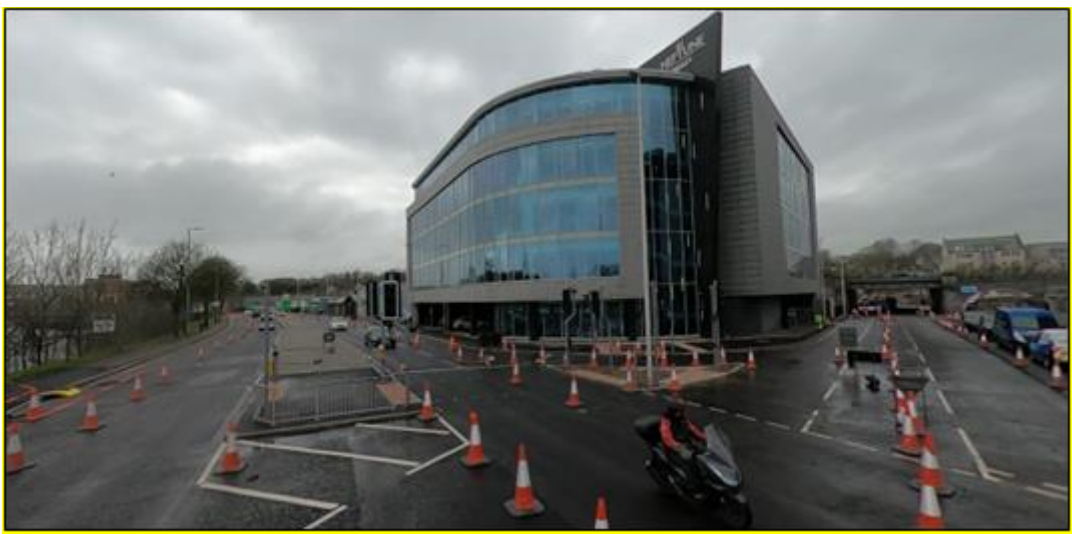
North Esplanade West looking toward Palmerston Place West April 2023
