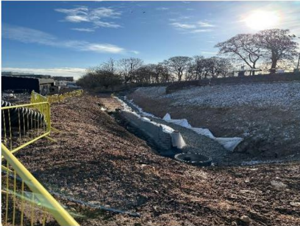
Grid Line 1 retaining wall
